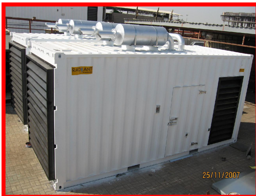
2 x 1500 kva containerized silent gensets powered by PERKINS Engines Model 4012-46 TAG 2A
